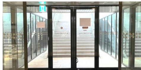
② If you go up the stairs, there is an exit door to outside.
